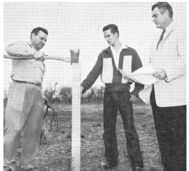
Plans for things to come...Stanley Clayton, far right, superintendent at North East School District in 1955, helps drive the first stake signaling the beginning of construction at a new school.
